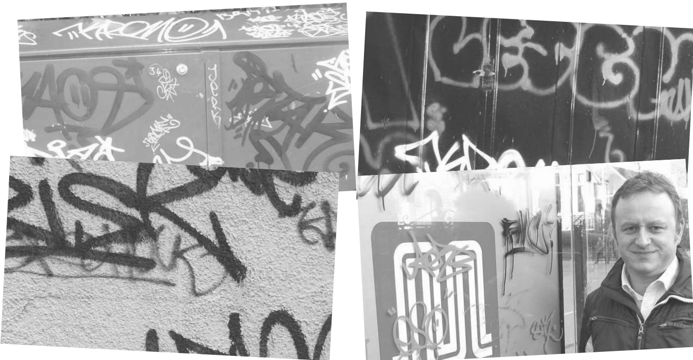
Councillor Tim Pickstone with just a small amount of Graffiti that local residents have complained about in recent months.
